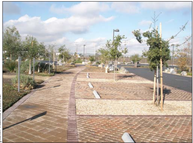
Parking spots with permeable pavement.
