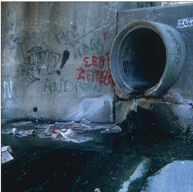
Stormwater runoff often discharges to local waterbodies and can carry a variety of pollutants from roads, parking lots and other areas.
