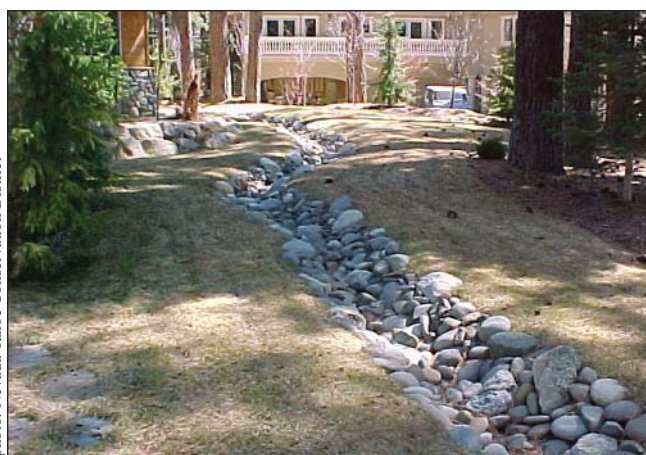
Rocklined swales are a natural way to convey runoff.
